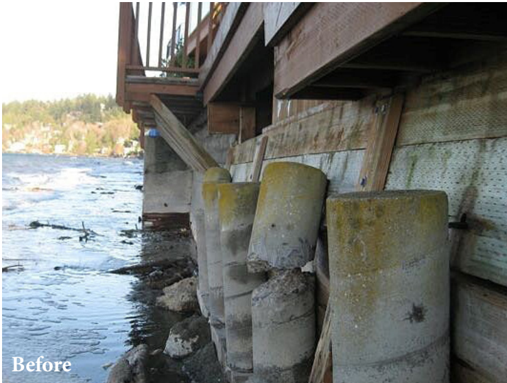
Removing shoreline bulkheads to improve fish habitat. Native vegetation, wood structures, and other natural shoreline protection elements are installed to prevent erosion from wave action. (King Conservation District)
