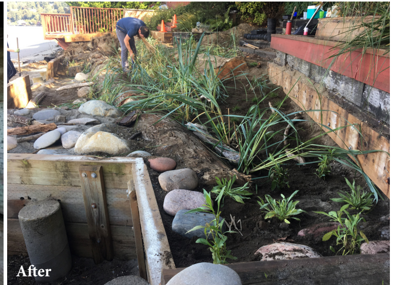
Removing shoreline bulkheads to improve fish habitat. Native vegetation, wood structures, and other natural shoreline protection elements are installed to prevent erosion from wave action. (King Conservation District)
