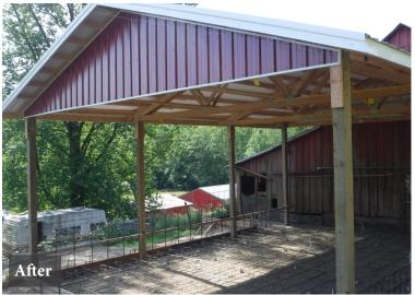
Constructing roof structures and stable, non-eroding surfaces in areas heavily used by livestock. This helps prevent mud and animal waste from reaching waterways, which is especially important during rainy seasons. (Kitsap Conservation District)
