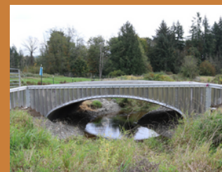
Removing fish barriers and replacing them with bridges that allow fish access.
