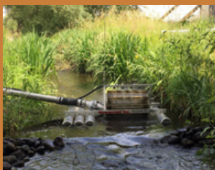
Installing fish-friendly screens on irrigation intakes.
