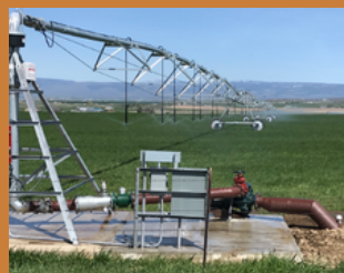
Upgrading irrigation systems to more efficient sprinkler systems.
